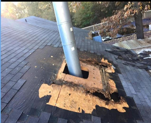
Complete tear down and re-build of the chimney frame around the flue pipe. Install new OSB walls and a underlayment. Install new chimney flashing and cover flashing with underlayment, then wrap chimney with a moisture wrap and install new vinyl siding trim, corners and panels on chimney. Install new shingles to best color match existing roof system. Clean up all trash from project and remove from property.
