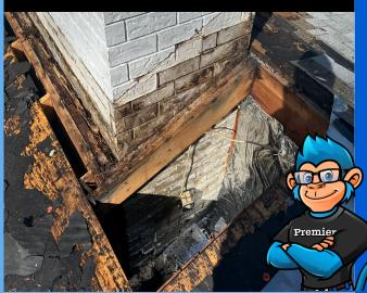
We Completely tear off the shingles and any old flashing around the chimney. Then we inspect and replace any bad wood found on the roof system. Next we install new roofing underlayment and new custom made chimney flashing and seal. Next we install new shingles to match your existing roof system and clean the work area. Last we remove the project trash and remove from property.
