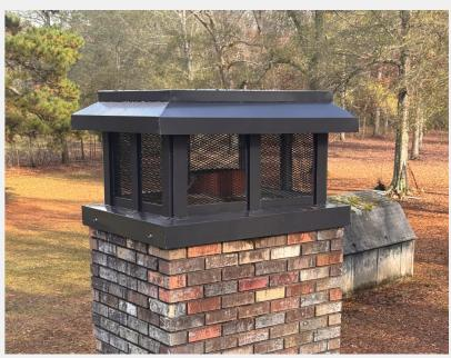
Every detail of the Royal Cap is intentional: its raised architectural roof-line improves draft performance, enhances smoke escape, and prevents heat trapping inside the chimney. The expanded metal screening blocks birds, rodents, and debris without restricting ventilation. Each unit is mechanically fastened, sealed, and built to outlast every traditional store-bought or builder-grade chimney cover on the market.
